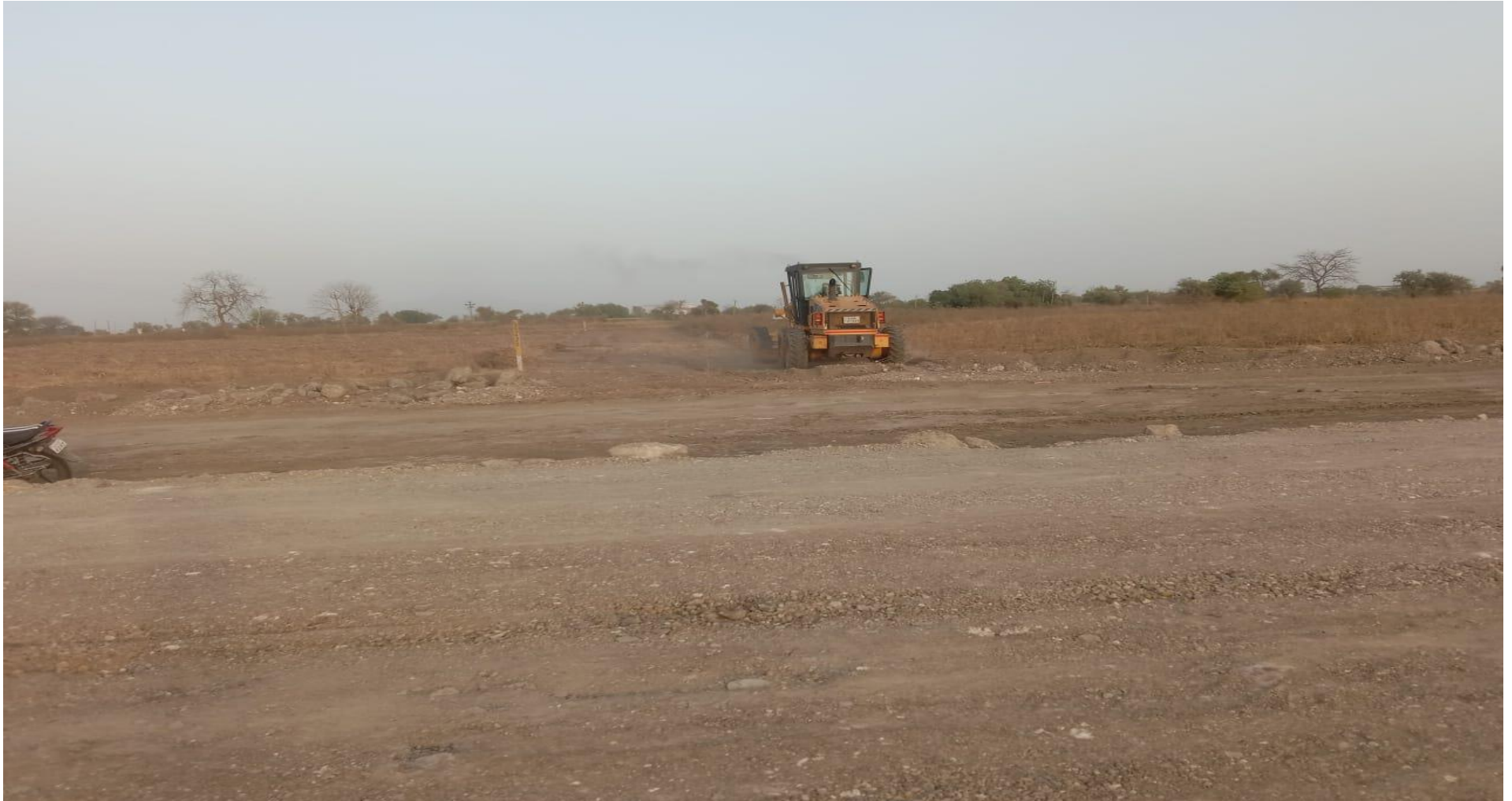
Cleaning and Grubbing wor progress at project site
