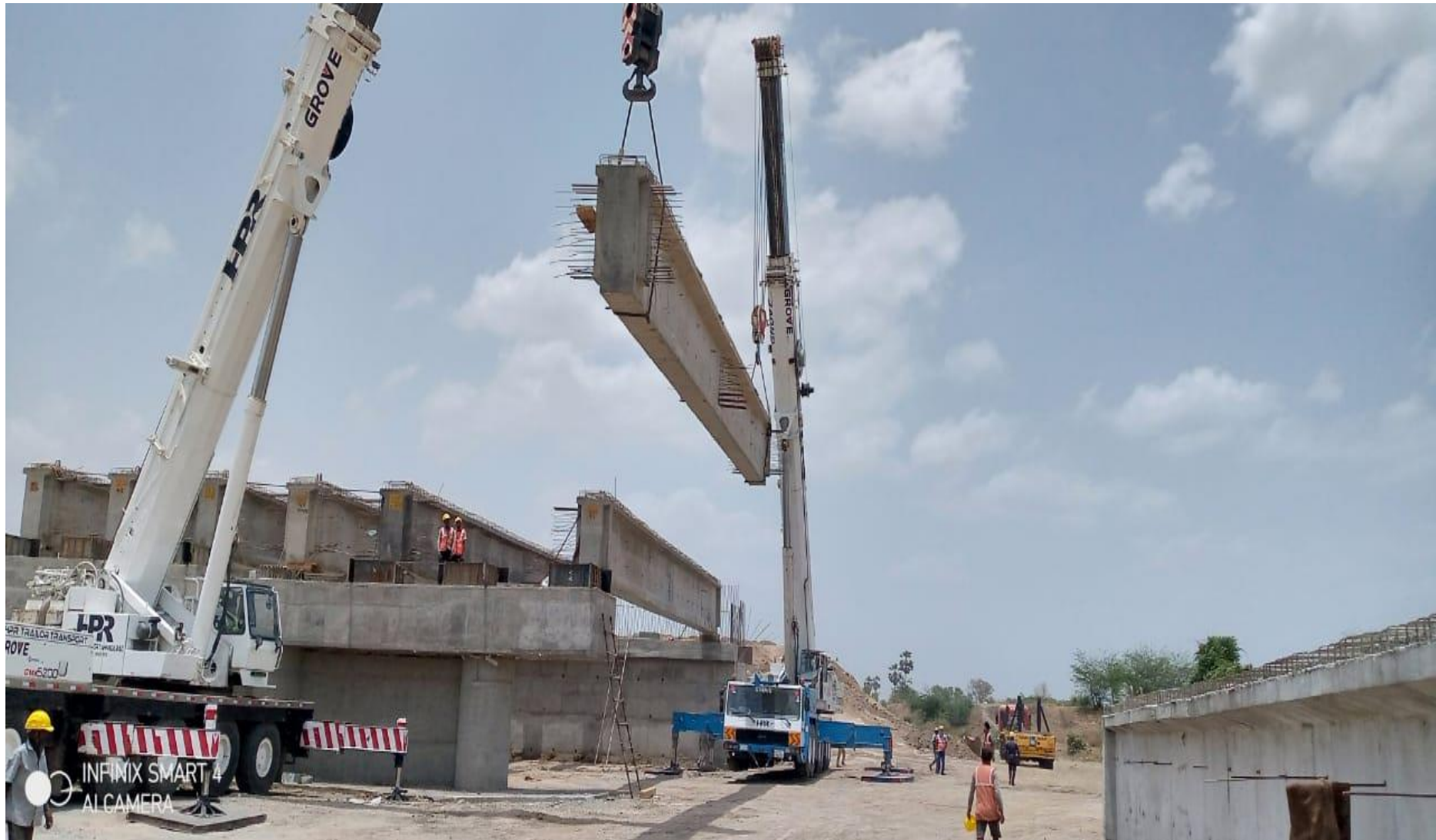
Girder launching at Major Bridge Ch-359+936
