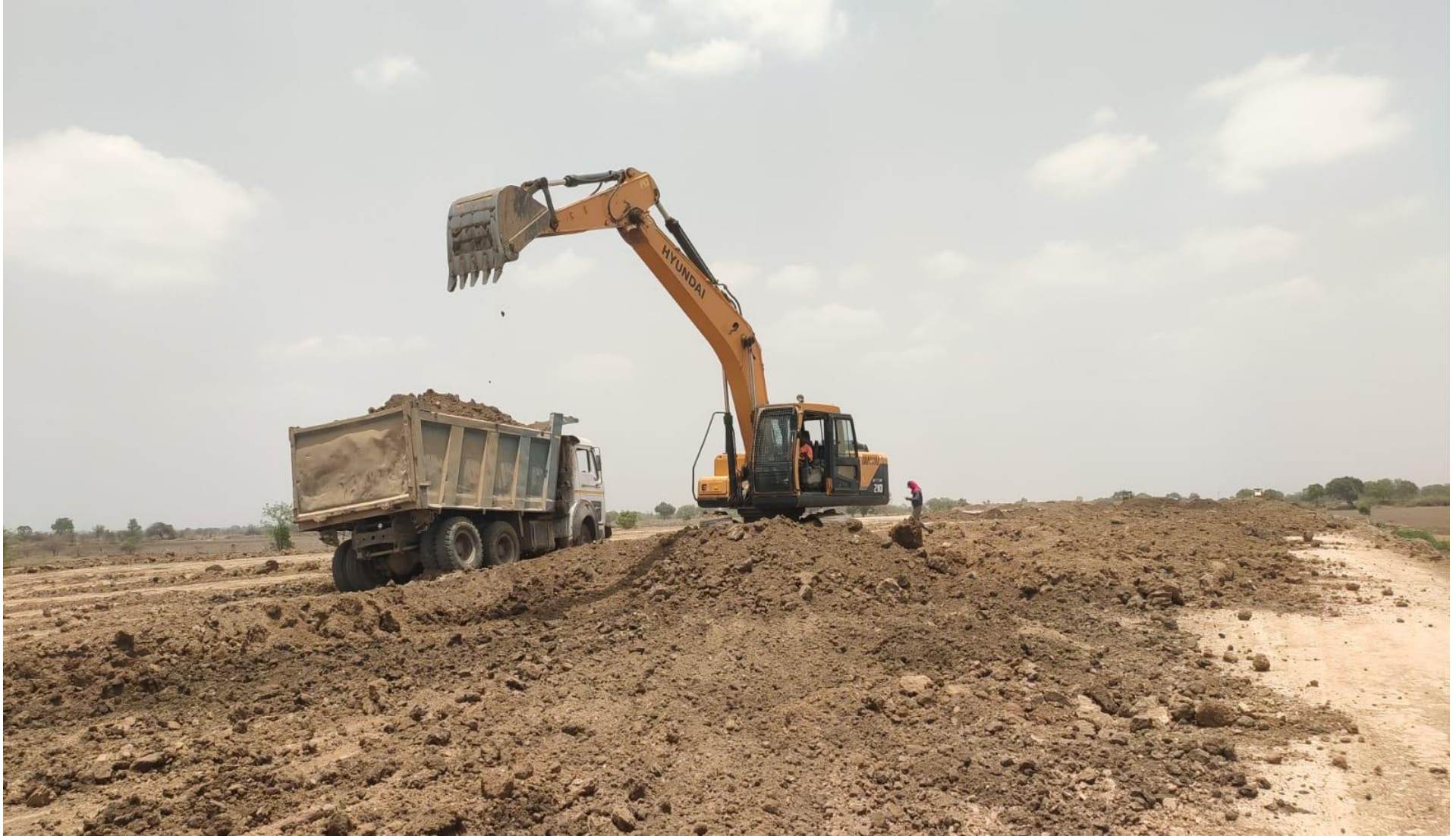
Black cotton soil removing at site
