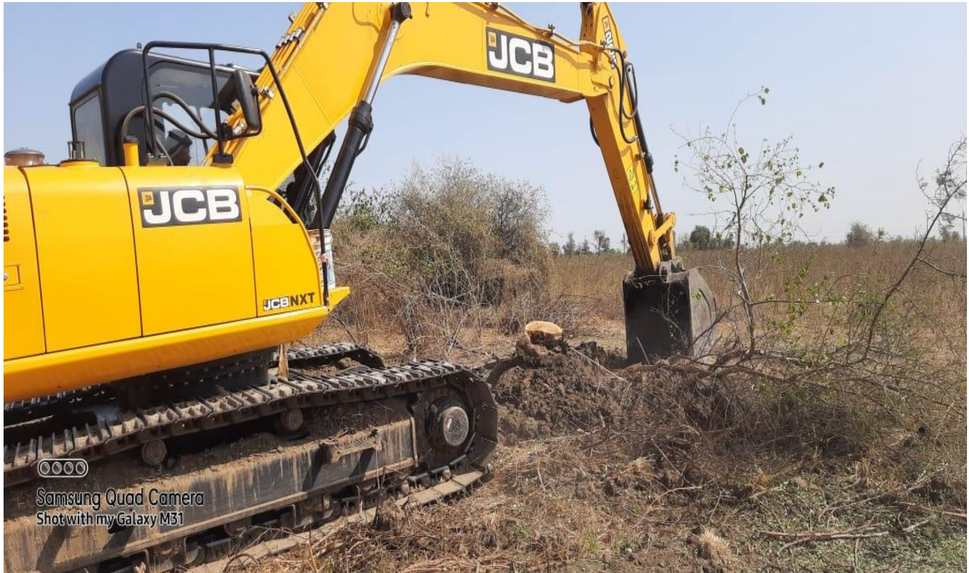
C&G work and Roots removal in progress
