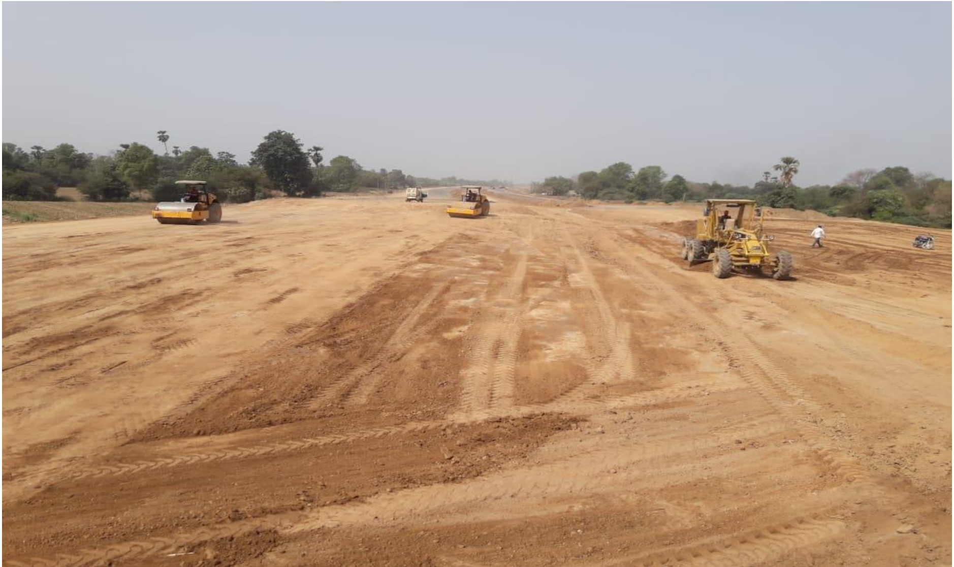
Embankment Layer in progress
