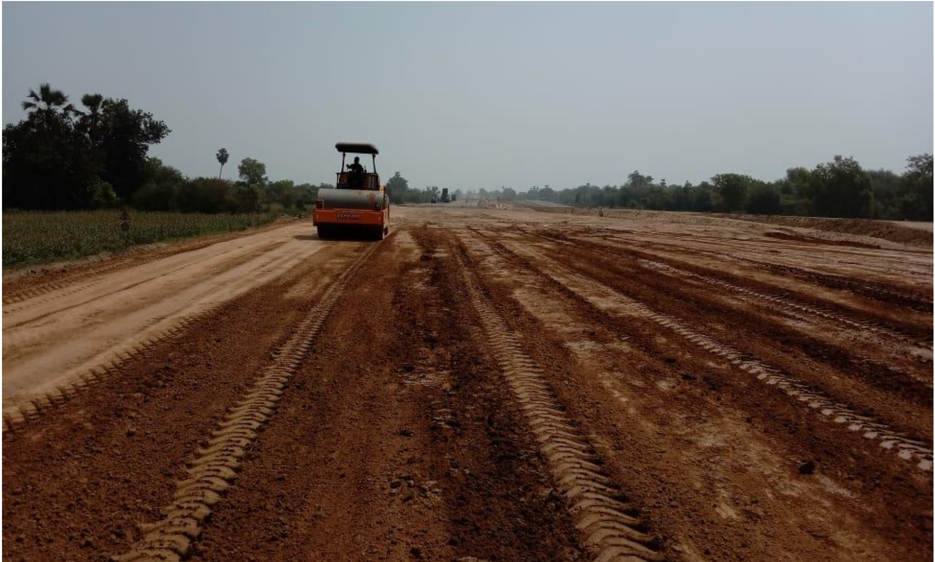
Embankment Layer in progress
