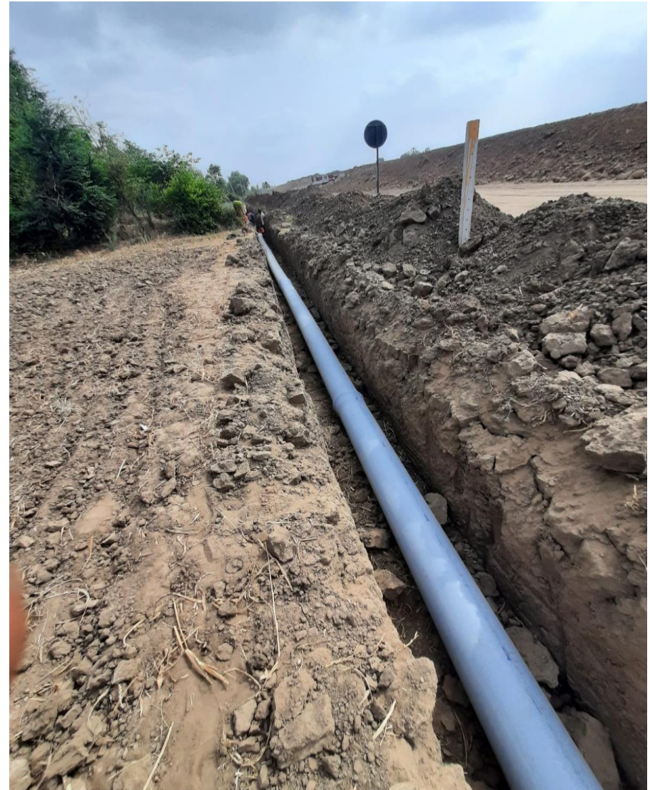
UGPL pipe laying work in progress 356+700 rhs
