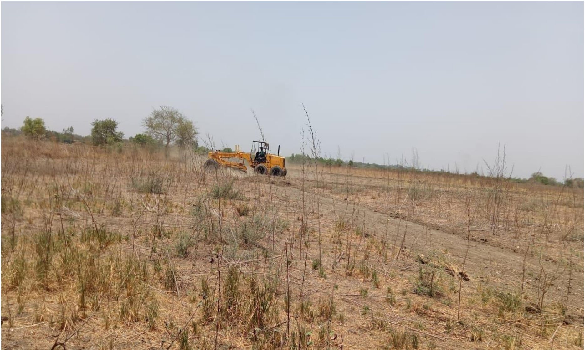
C&G work in progress at ch.363+310
