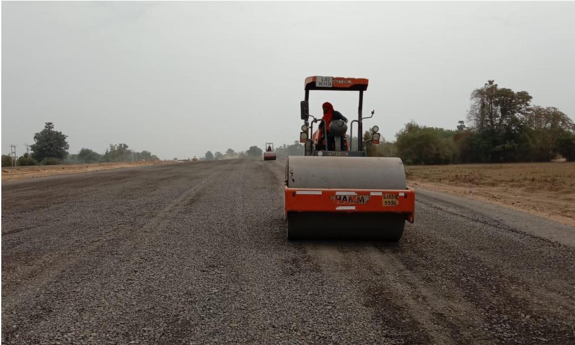
GSB Top Rolling in progress
