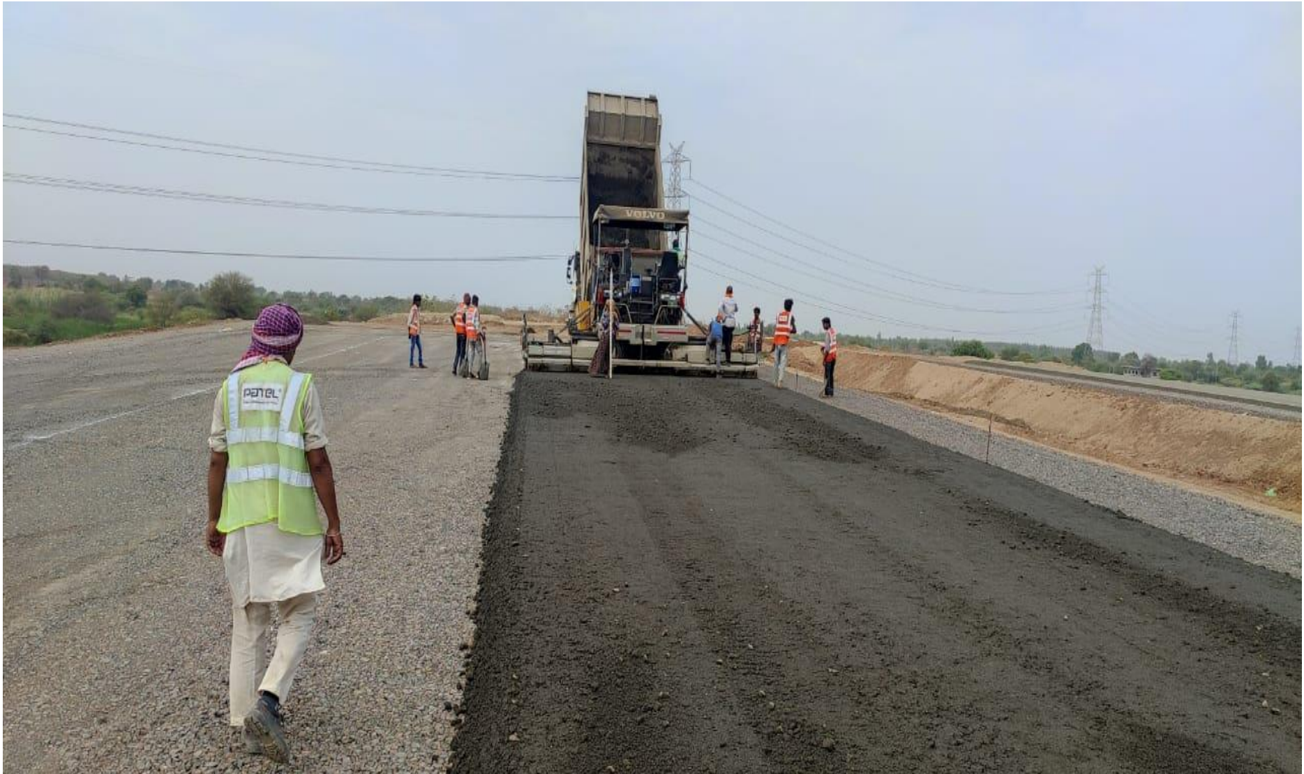
WMM laying in progress
